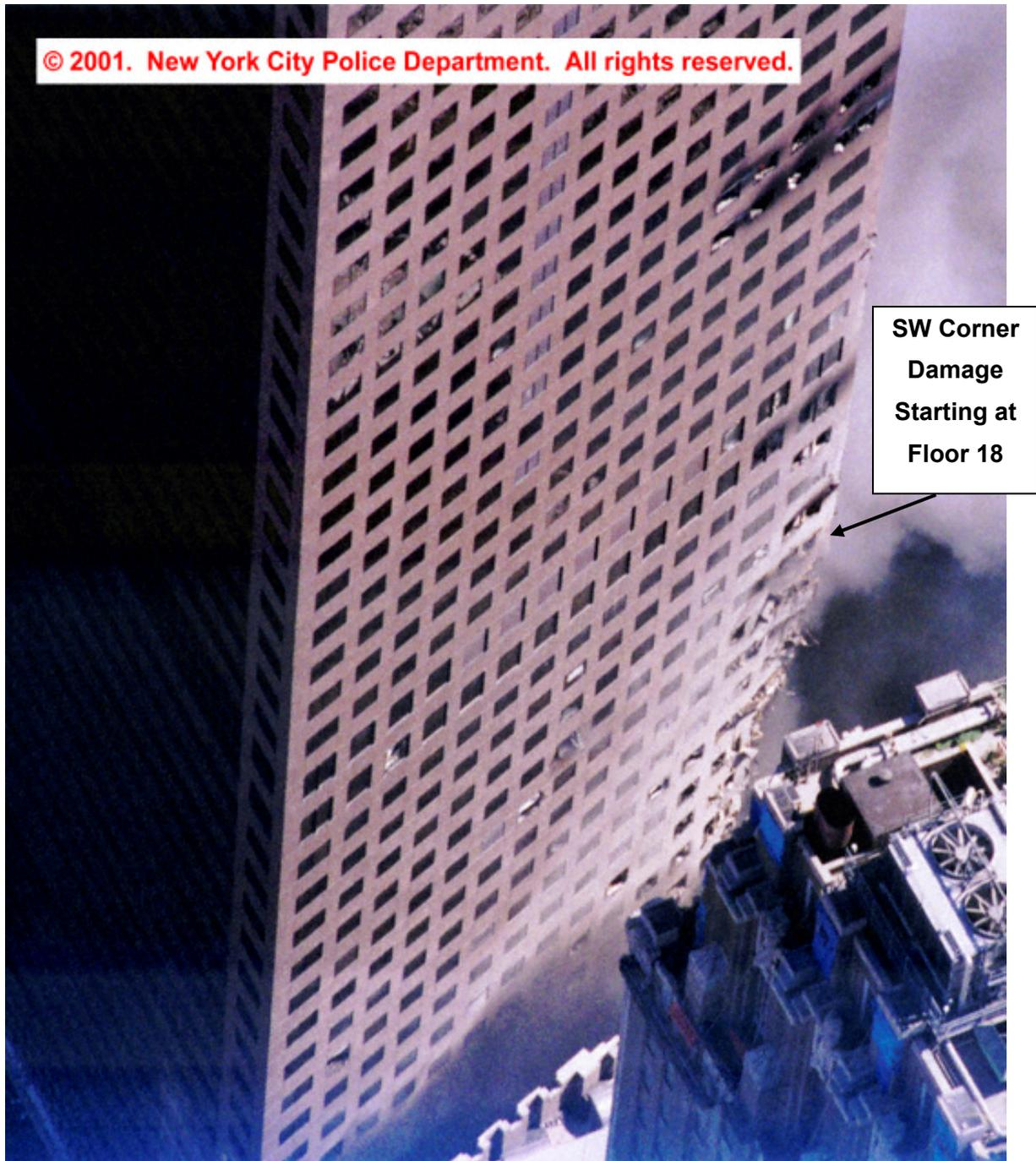
Figure L-22a. Debris damage around Floor 18 of the southwest corner.
