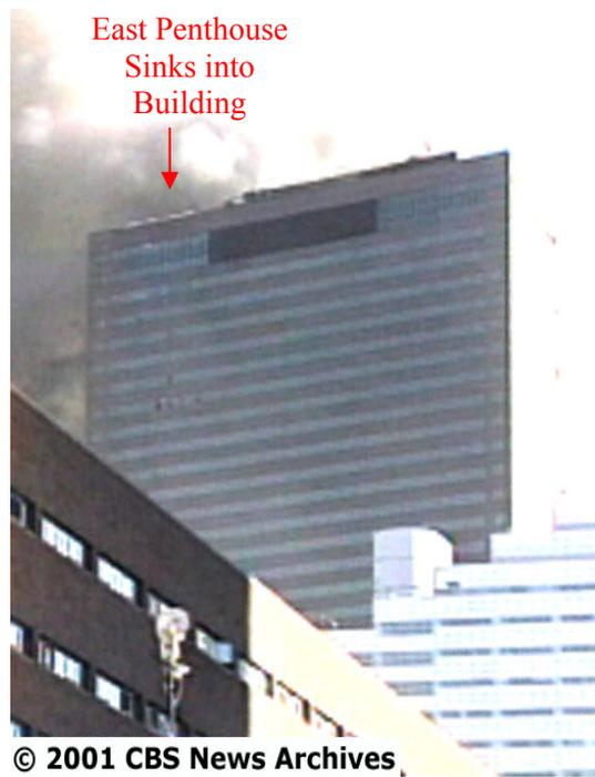
Figure L-26. East penthouse sinks (2.2 s).
