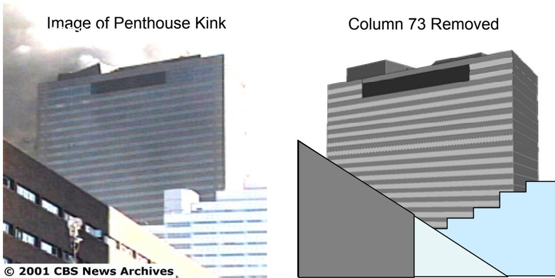
Figure L-41. Geometry changes for removal of column 73.
