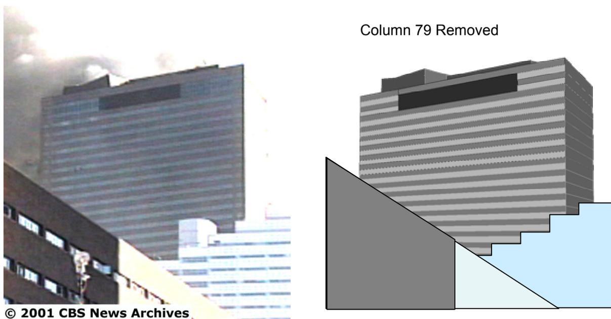
Figure L-45. Geometry change for removal of column 79.
