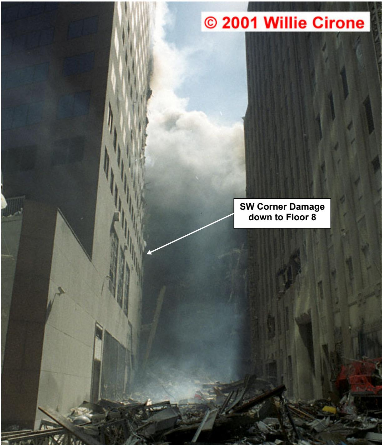
Figure L-22b. Debris damage around Floor 8 of the southwest corner.
