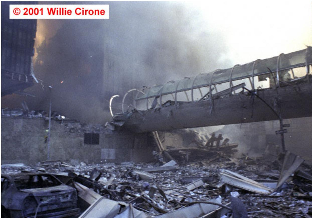
**Figure L–23a. Pedestrian bridge and debris on Vesey Street after WTC 1 collapsed.**
