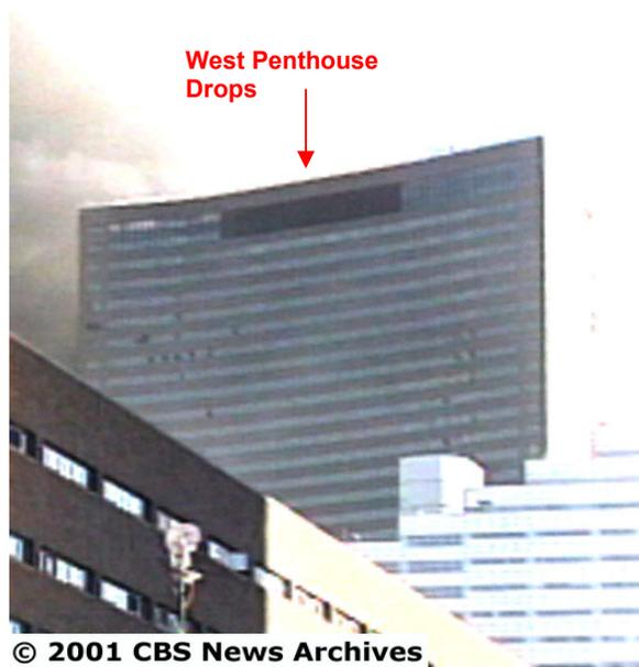
Figure L-27. Center screenwall and west penthouse sink (7.9 s).
