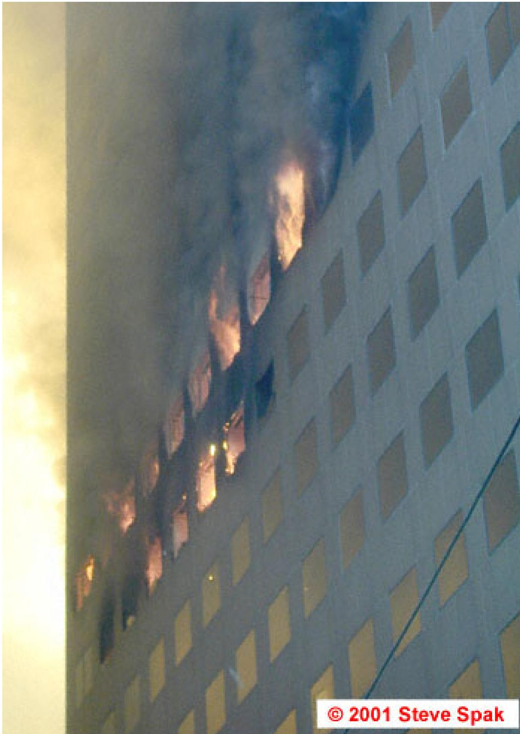
Figure L-24a. Fires on Floors 11 and 12 on the east face.
